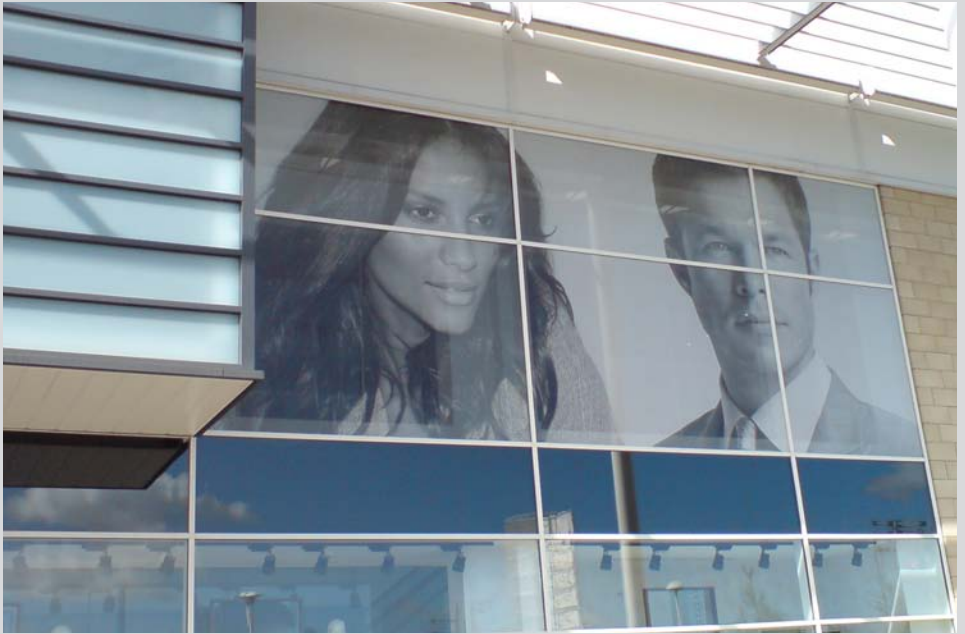
_ project: _ next brent cross
